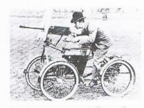
The Simms Motor Scout was the first armed, petrol engined vehicle ever built. Simms built the vehicle by mounting a Maxim machine gun on the front wheels bar of a De Dion-Bouton quadricycle. He also put an iron shield in front of the car for the driver's protection. The driver also operated the machine gun.
